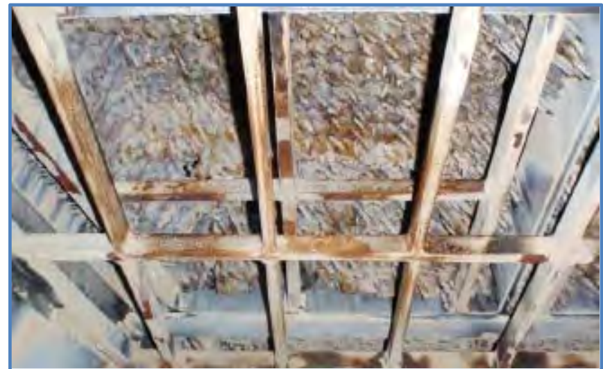
Brominated PAC - Upstream Injection
